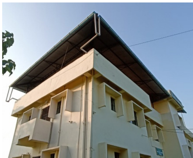
Rain Water Harvesting unit by KVK-Thoubal
