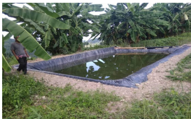
Water harvesting structure "Jalkund": KVK Phek
